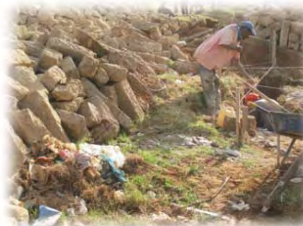
AIDS clinic construction
